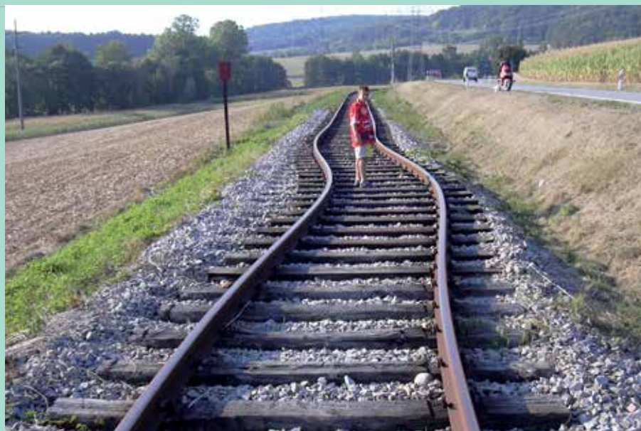
When thermal expansion becomes a hazard (photo: ulrich-rapp.de)
