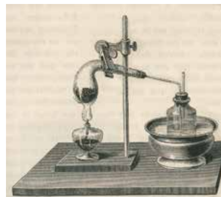
Hardly changed from the times of the ancient Egyptians — production of ammonia spirits from animal bones; from Stöckhardt, The School of Chemistry (1863)
