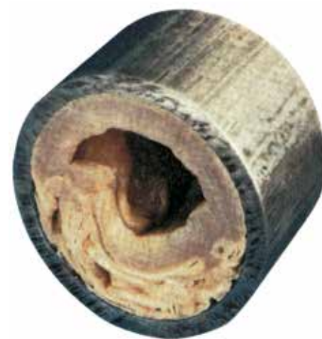
A water pipe narrowed by calcium deposits (photo: ELGA Berkefeld GmbH)
