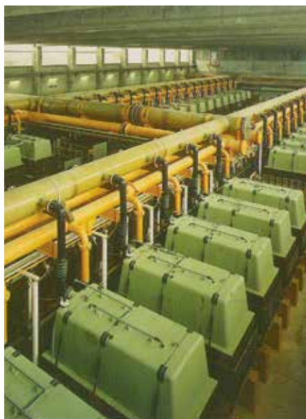
During chloralkali electrolysis, chlorine, hydrogen, and soda lye are produced (photo: Lurgi).
