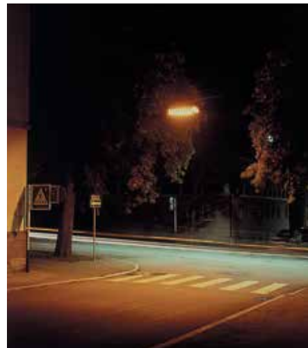
Sodium vapor lamps provide plenty of lighting on pedestrian paths, even in gloomy weather.
