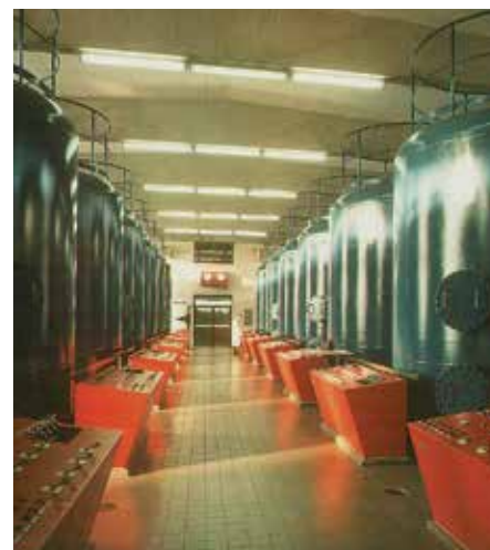
Fine-cleaning of drinking water with activated charcoal (Lurgi factory photo)
