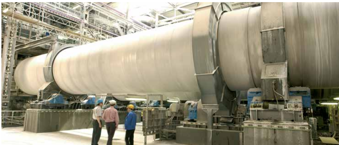
Steam-heated rotary furnace in which baking soda is converted into the final product — soda (photo: Deutsche Solvay-Werke).
