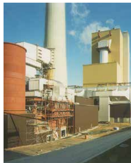
Facility for the desulfurization of flue gas (photo: Lurgi)
