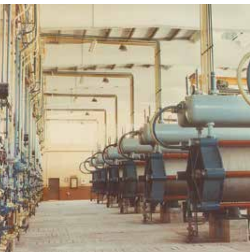
Industrial hydrogen production by the Lurgi pressure electrolysis process (Lurgi factory photo, Germany)
